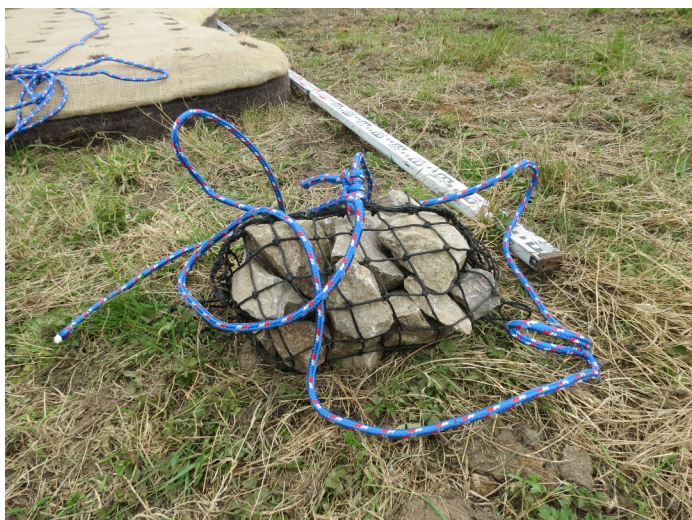
Anchors of netted rocks are then tied to loops run through the substrate mat. The ropes anchoring the islands are cut to the length required, ensuring enough slack to account for natural rises in water level.
